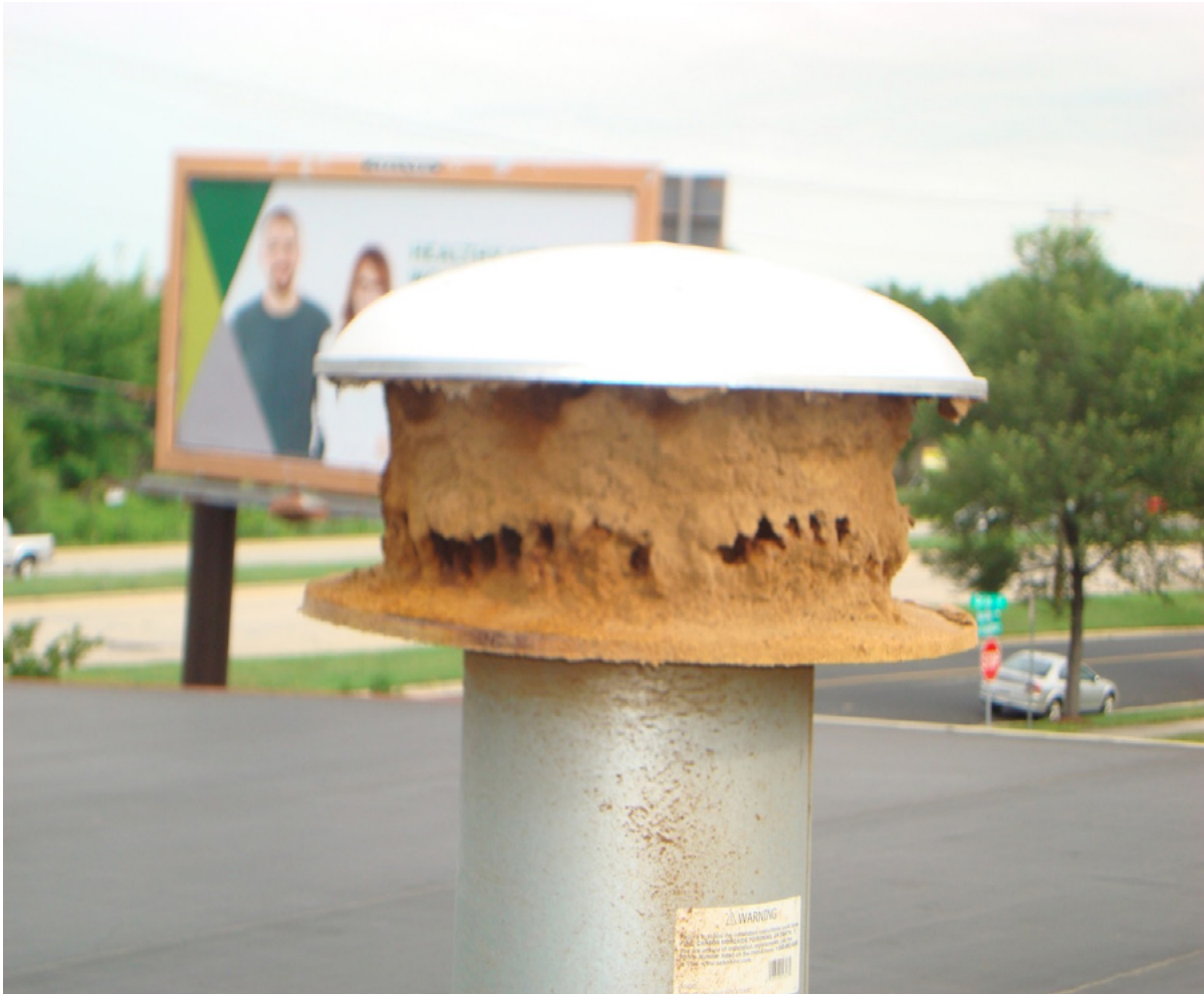
Figure B1. Roaster exhaust stack plugged with chaff residue and debris, NIOSH ventilation assessment, July 2015.
