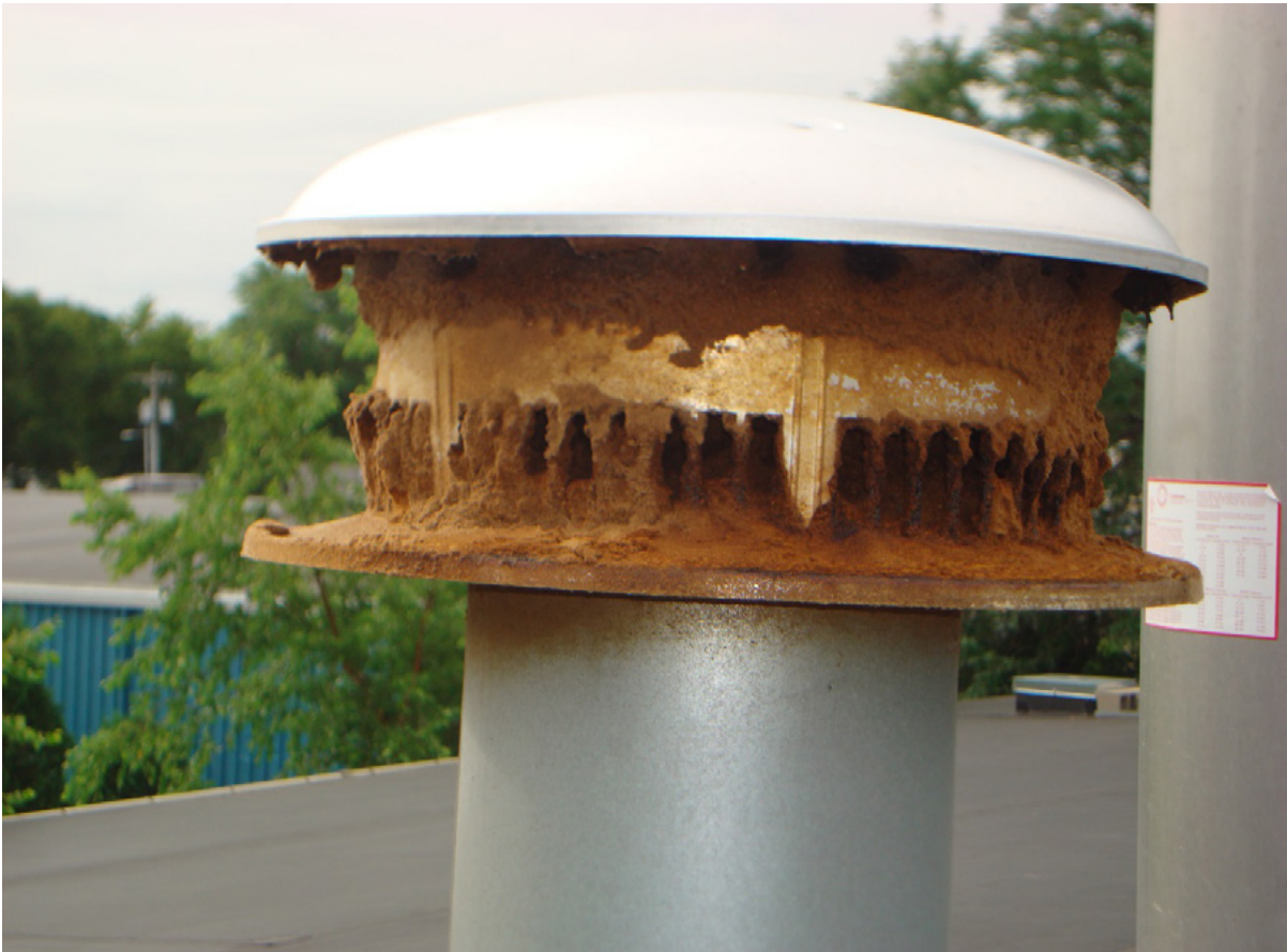
Figure B2. Other roaster exhaust stack plugged with chaff residue and debris, NIOSH ventilation assessment, July 2015.
